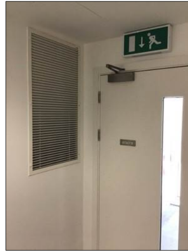
Example fire door with excessive gap at the top.
